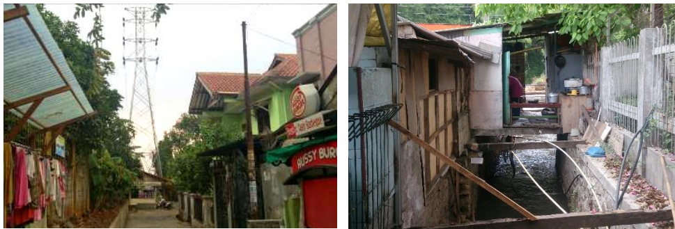
Figure 9. Violations of areas reserved for utilities. Residential area under high voltage electric lines (left). Expansion of buildings above waterways (right).
