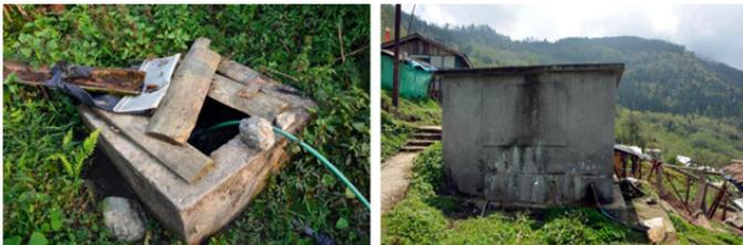
**Figure 5.** Water from local springs are collected in storage well and subsequently supplied to the village tanks
