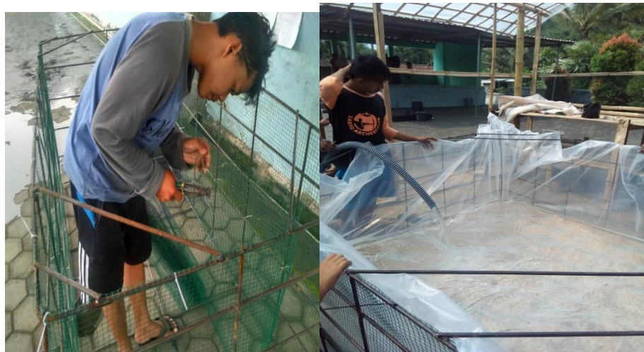
Figure 6. Making pond frames in the herbamina system
