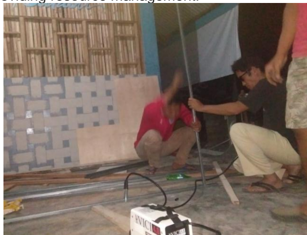
(b) steel frame welding of RUBAH
