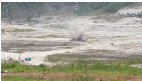
Figure 5. Blasting Activity PT. Semen Baturaja (Persero) Tbk
