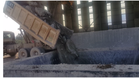
Figure 7. Dumping Activities at the Crushing Plant
