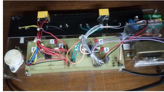
Gambar 9. Fire Sensing System
