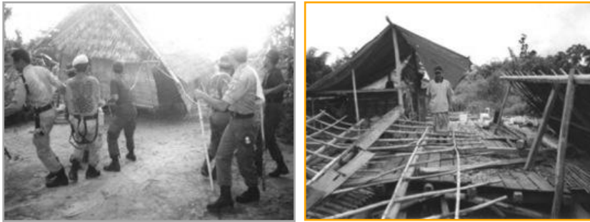
Figure 11. SapuJagat Tim demolishes a Moronene house in Hukaea Village (left); a Moronene man looks at ruins of his house (courtesy: Suluh Foundation)
