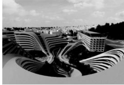
Gambar 5 Beko master, Belgrade – Zaha Hadid Organic Curves – Deconstructivism Sumber : Zaha Hadid Architec.com
