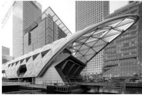
Gambar 15 Geometric Shape Hybrid Organic curves with space frames Canary wharf,UK – Norman Foster Sumber : Arcspace.com
