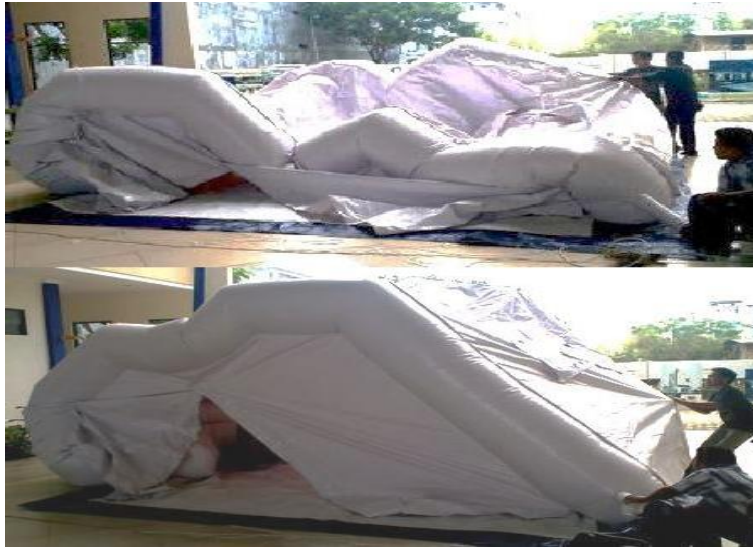
Gambar 2. Proses Setting-Up Portable inflated Structure
