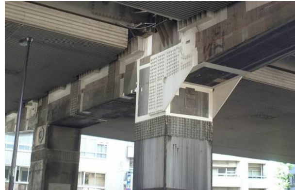
Figure 4. Steel Frame Pier with Fatigue Retrofit Work
