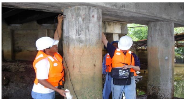
Figure 7b. UPV Test on Column C2
