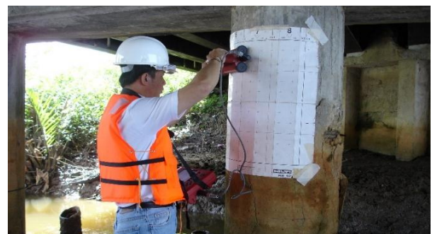
Figure 9a. Pachometer Survey on Column C3
