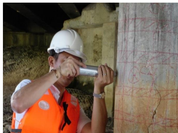
Figure 6. Rebound Hammer Test on Column C3
