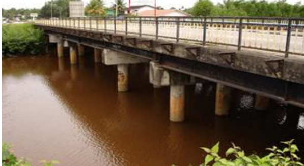
Figure 1a. Bridge General View
