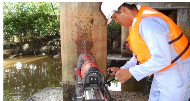
Figure 9b. Core Sample Extraction on Column C4
