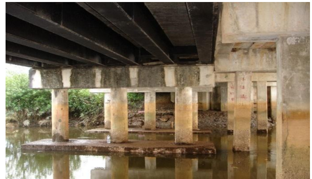
Figure 1b. Bridge Underside View
