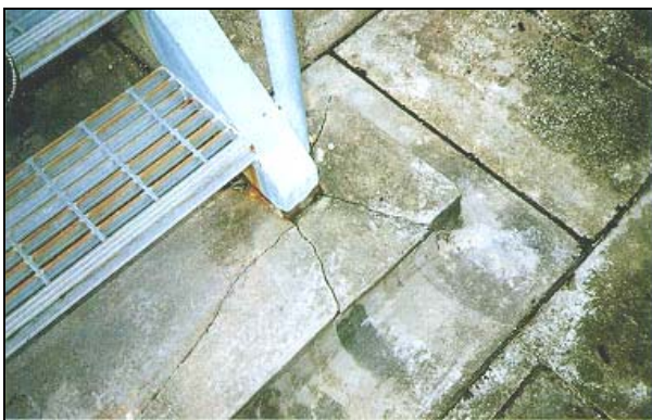
Figure 5. Support cracking [3]
