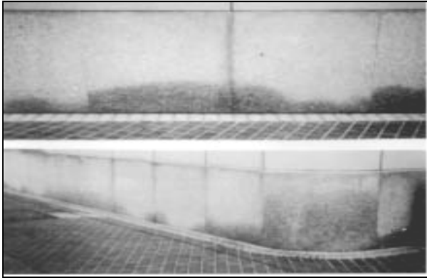
Figure 13. Water penetration [1]
