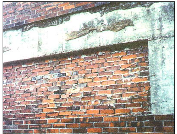
Figure 7. Cement oozing
