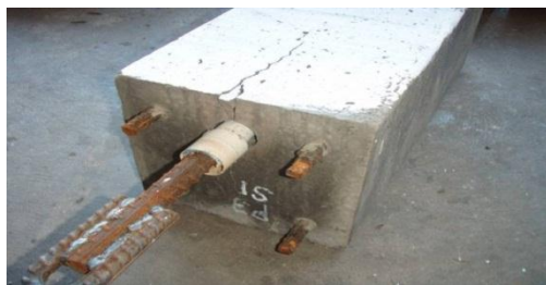
Figure 2(a). Failure of Geopolymer Concrete Specimen
