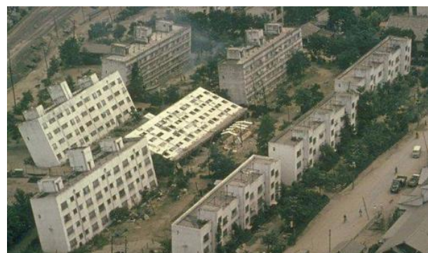
Figure 1. Liquefaction due to Niigata Earthquake [2]
