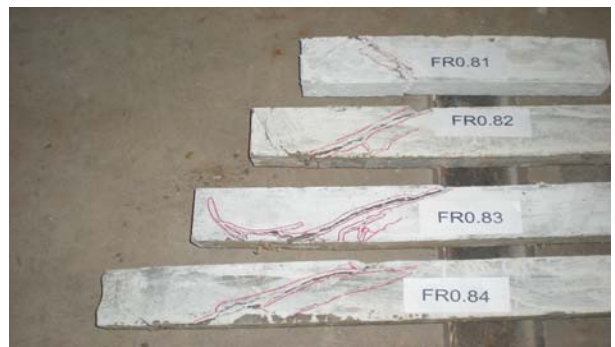
Figure 10. Cracking patterns HSFRC beams with 0.8% fibers for a/d = 1, 2, 3 and 4
