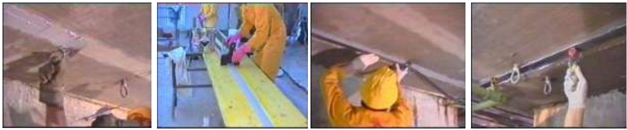
Figure 4. Application CFRP Plate
