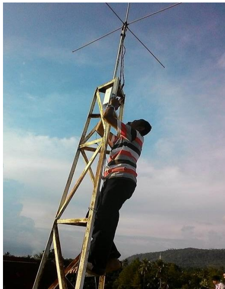
Gambar 5. Pemasangan base station
