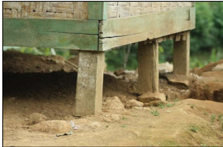
Figure 8: House on Stilts Constructions
