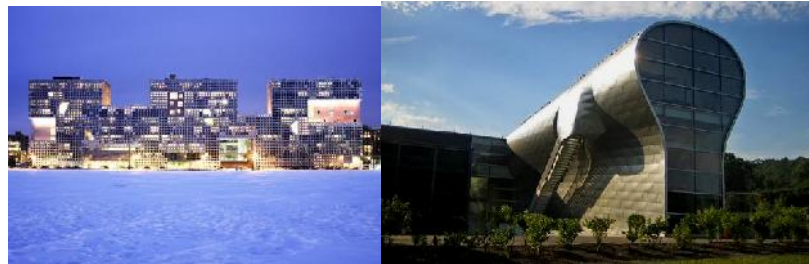
Gambar 5. Kiri: The Simmons Hall Dormitories,
