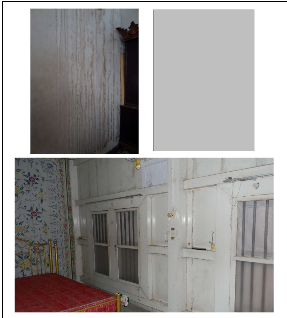
Gambar-18: Dinding kayu
