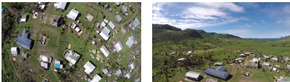
Figure 3. Nokonoko Village Damage Source: Field survey
