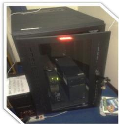
Gambar 8. Mekanik- Rak Server Raja Rack 19 Wallmounted 8u 500mm
