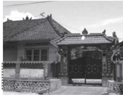
Figure 8. The New Gate Applying Traditional Style and Old Wall Applying Modern Style Shows the Process of Transformation in Kamasan
