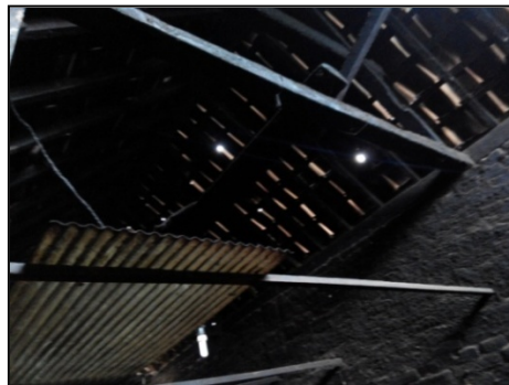
Figure 4 Condition of Ceiling
