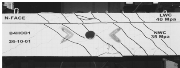
(b) Crack pattern of specimen B4HOD1
