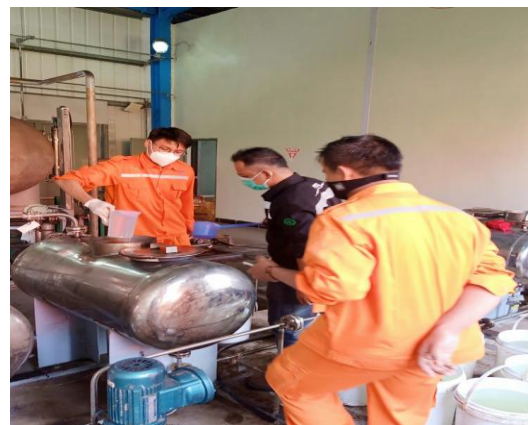
Figure 4. Electrolyte Replacement Process
