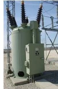
**Gambar 6.** OCB (Oil Circuit Breaker)
