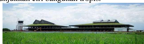
Gambar 4. Atap Terminal Bandara Banyuwangi
