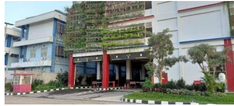
Gambar 7. Green Fasad Terminal Joyoboyo
