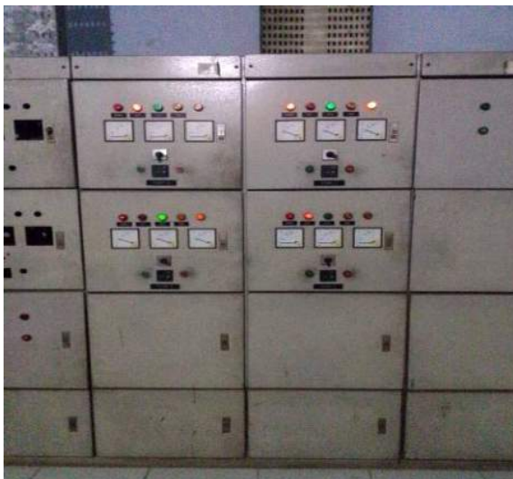
Gambar 21. Panel Star Delta di PDAM Tirta Musi Unit Pelayanan KM IV Palembang
