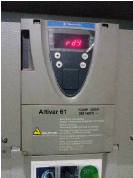
Gambar 18. Inverter di Unit Pelayanan KM4 PDAM Tirta Musi Palembang
