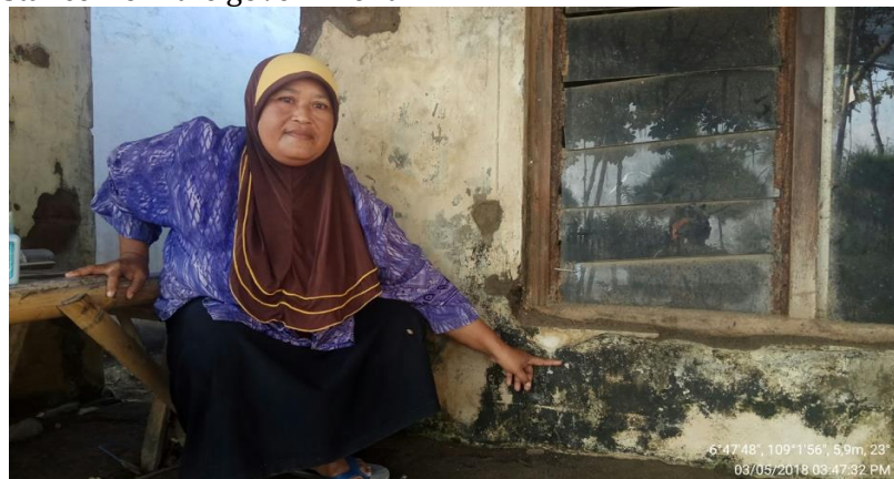
Figure 5. Weathered buildings due to tidal flood (Source: Field survey)
