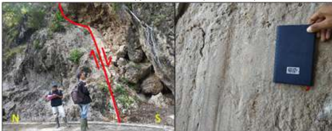
Figure 11. Normal Fault at Station SP1.6
