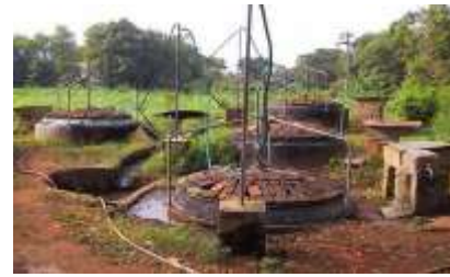
Gambar 4 Proses Penimbunan Digester ,Bak Control,Lubang Inlet,Lubang Outlet
