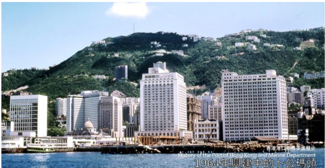
Figure 5. Blake Pier under Construction in 1964
