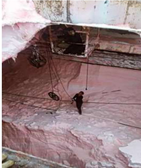
Figure 1. Wire out block repair
