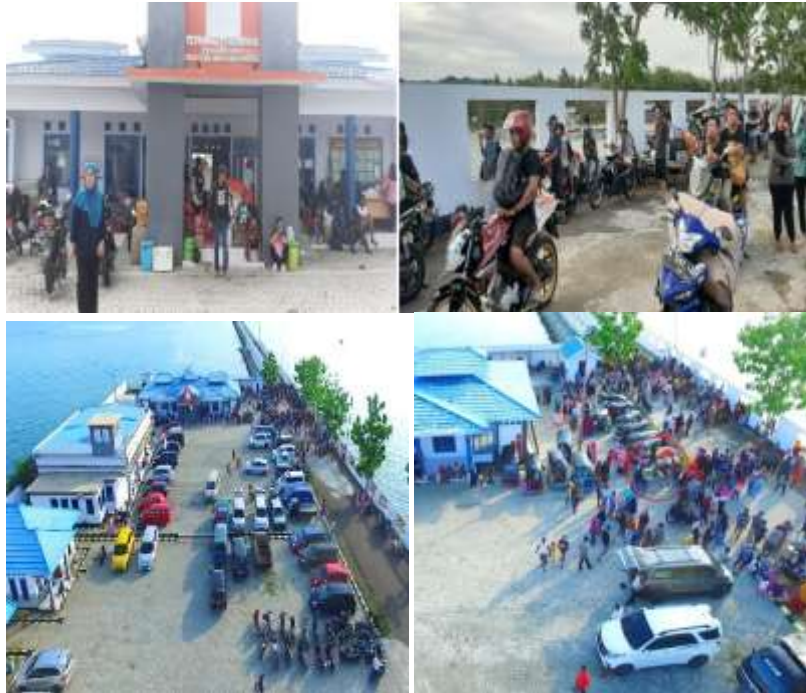
Figure 1 conditions Existing at the Marisa Ferry Terminal
