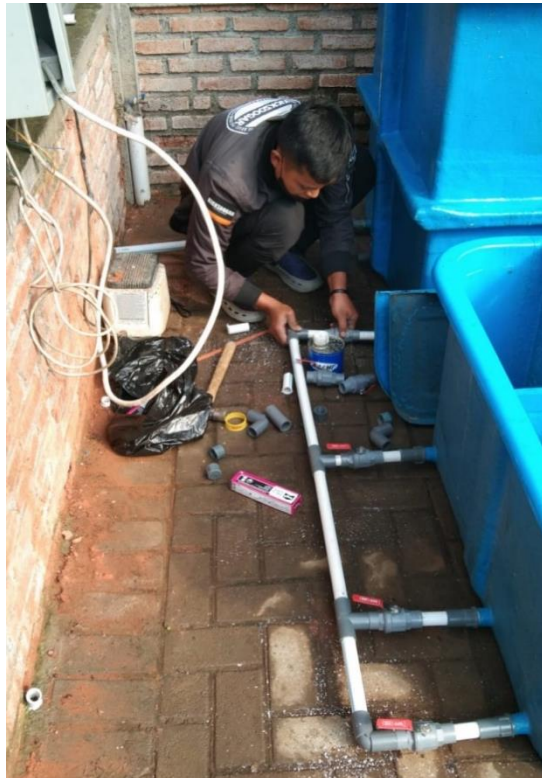
Gambar 3. Sistem inlet-outlet kolam
