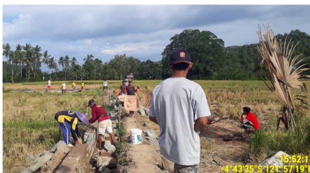
Picture 4. Irrigation channel works
