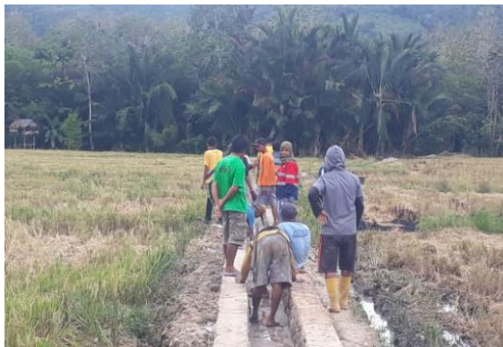
Picture 3. Assistance in Building Irrigation Canals
