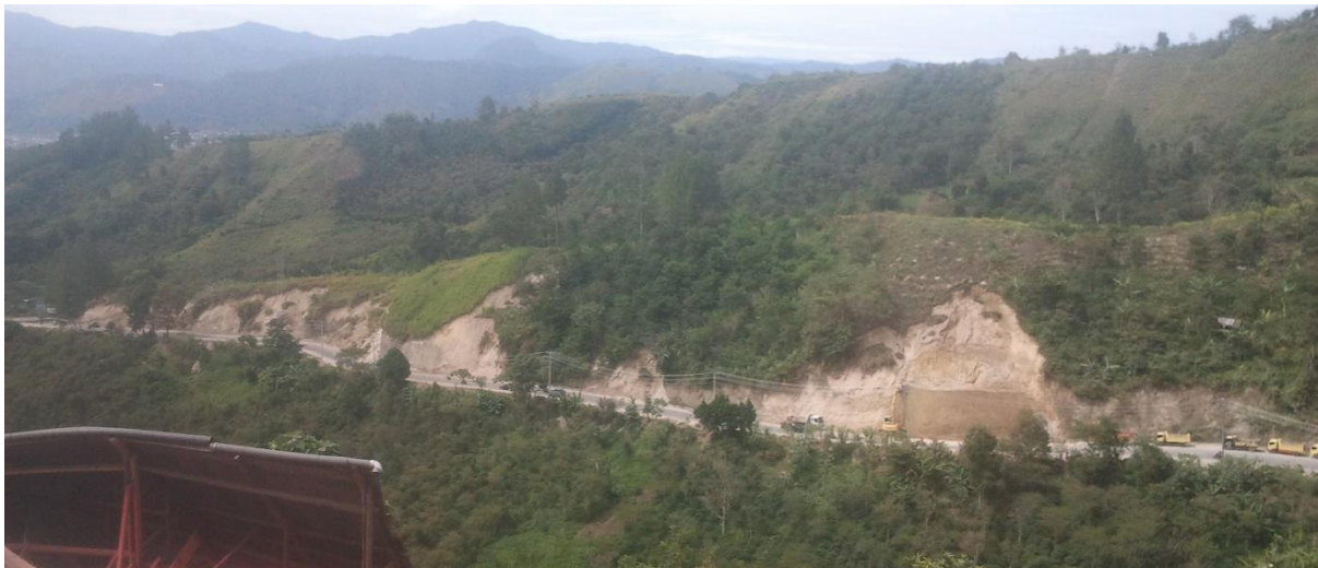
Figure 7. Landslide/slope failure along The Study area due to July 2 nd , 2012 earthquake
