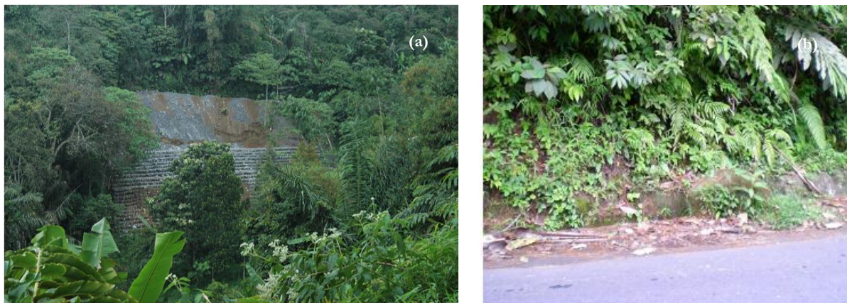
Figure 5. (a) The gabion and (b) Drainages built to prevent slope failure.
