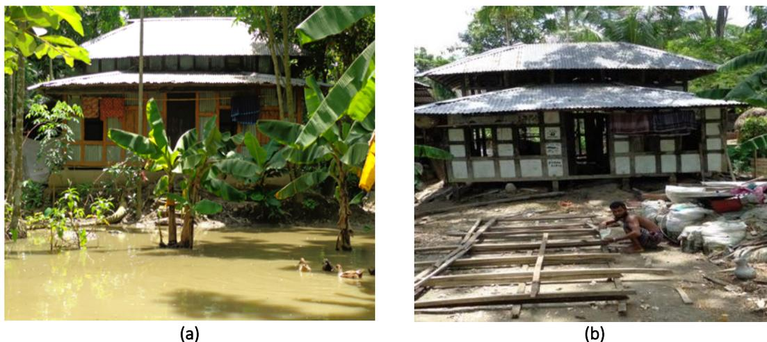
**Figure 16.** Flood and cyclone resilient housing system in Kazirchar village, (a) house built on raised land, and (b) house built on platform above the ground and basement.
