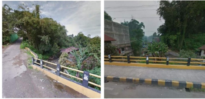
Figure 4. Existing Condition of Batang Agam River Upstream
