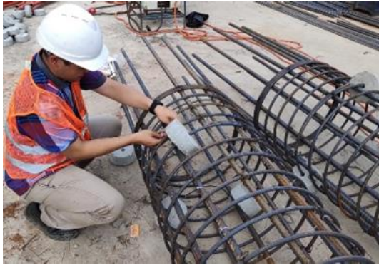
Figure 10 Fiber Optic Installation
