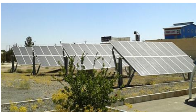
Figure 6. Using 20 kilowatts of solar energy for lighting part of the main campus of University of Kashan
