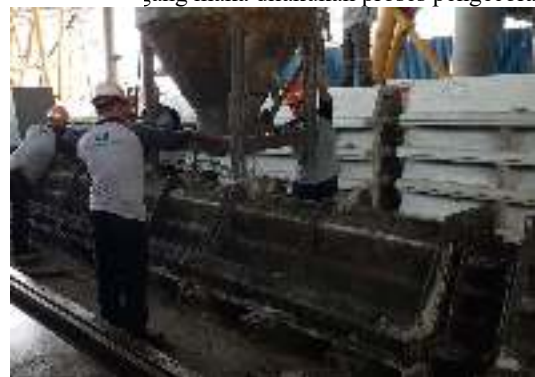
Gbr. 7 Proses pengecoran
