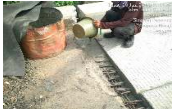
Gbr. 13 Pengecoran Joint Double Tee
