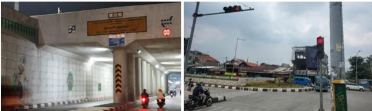
Figure 2. Underpass Condition and Simpang Bulak Kapal
