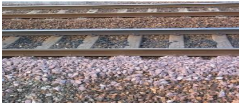
Figure 2. Granular material rail ballast
