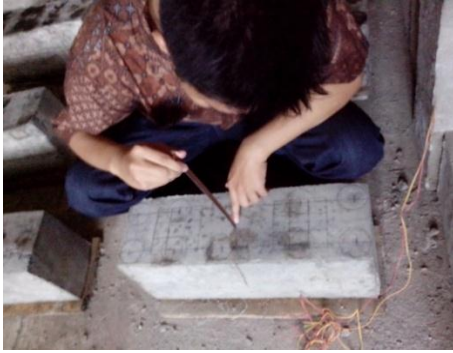
Figure 5. Measuring the actual crack depth
