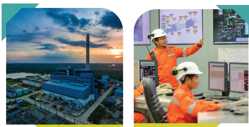
Figure 2. Operation & Maintenance Power Plant (O&M)
