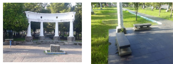
Figure 2. The Existing condition of Street Furniture (Source: Personal data)
