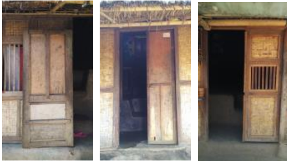
Figure 7. Several types of doors on bale Tani studied, still using bamboo, wood and bedek materials, with different shapes but still in the same design language. Source: Author, 2017
